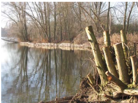
5. Coppiced willow in the foreground with recently completed spiling in the background.
