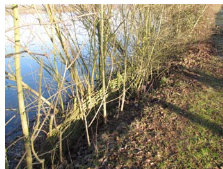
6. Mature spiling where the willow has sprouted and grown into a natural barrier.
