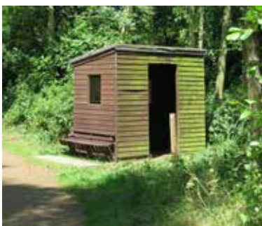
Bus Stop shelter
